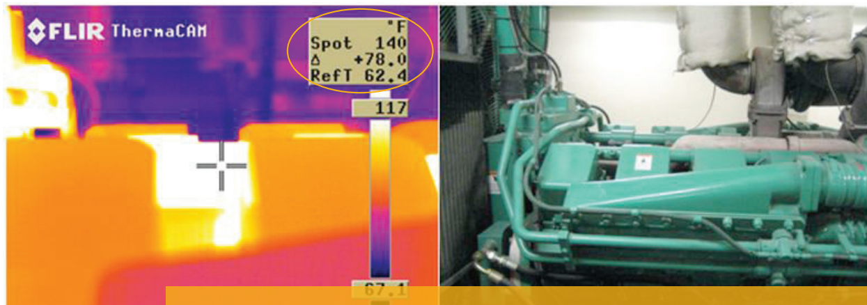
Figure 3: Generator A thermosiphon, thermal and normal image of top of engine, spot temperature 140°F
