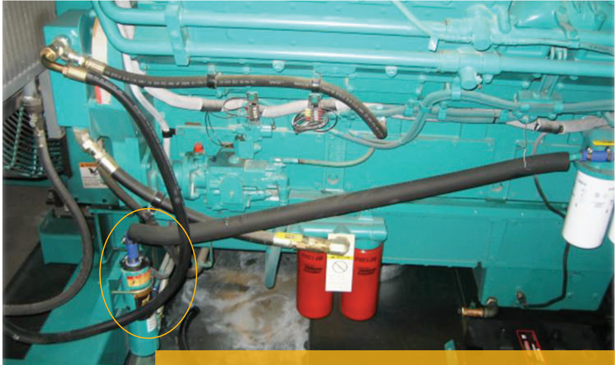
Figure 1: Example of thermosiphon engine block heater as installed on a typical standby generator.
